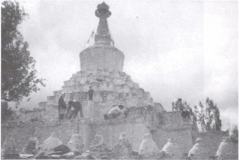
Plate XXVIII. The scene of pouring lime-water upon the clay plastered stūpa at Changspa.
