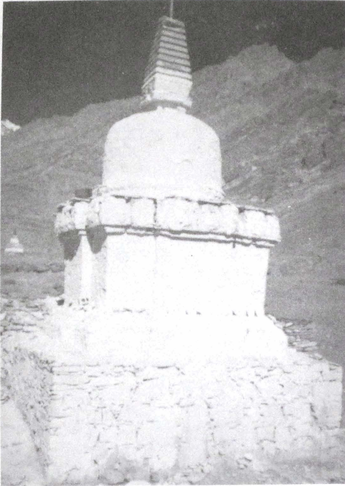
Plate XXIII. The Nirvāṇa stūpa having a low dome with pyramid-shaped umbrella-tower at Hemis valley.
